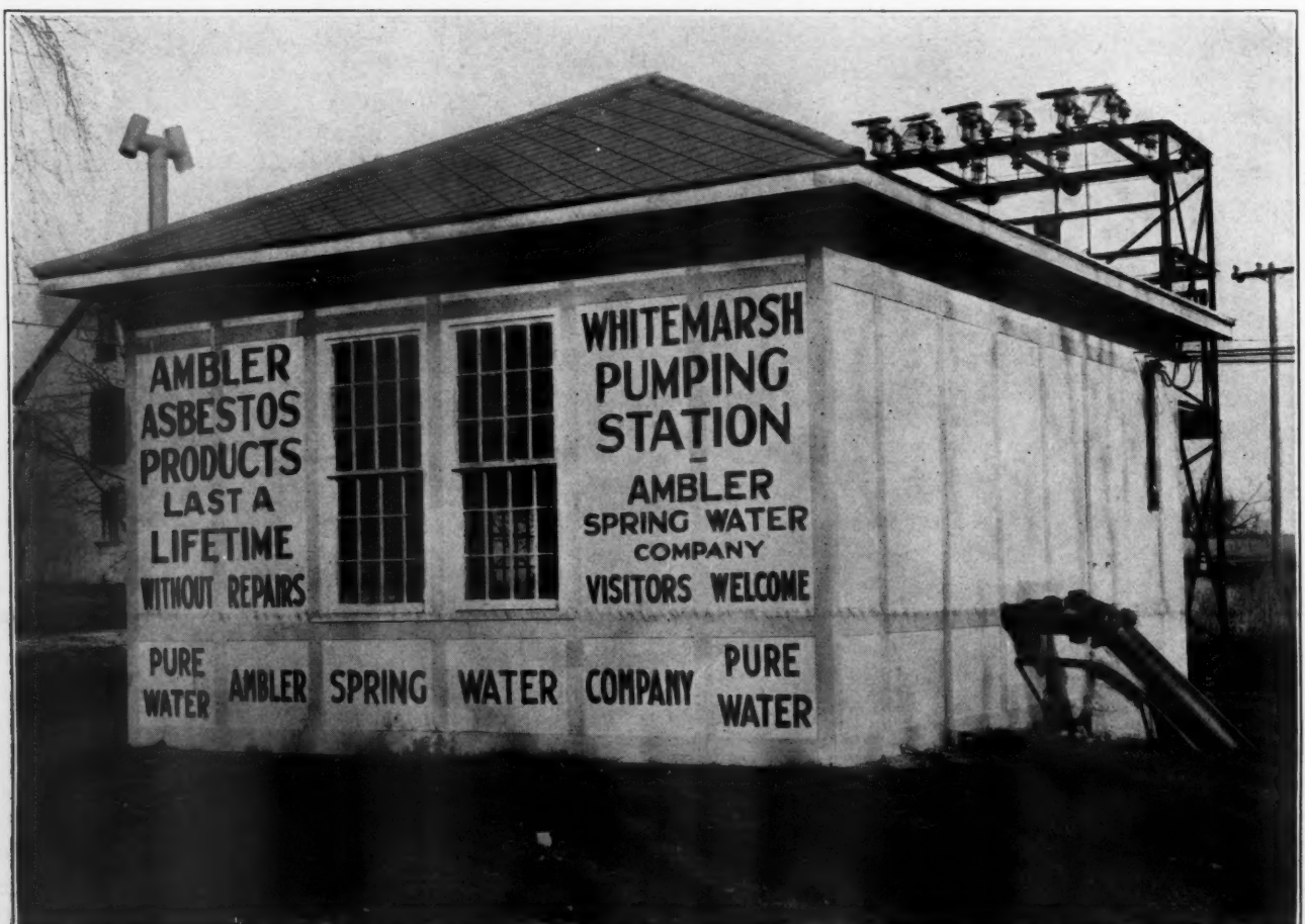
Pumping station which stands beside the quarry
